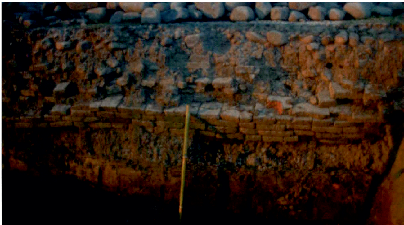
Fig. 1.7 (c): Exposed section showing the remains of brick structures
