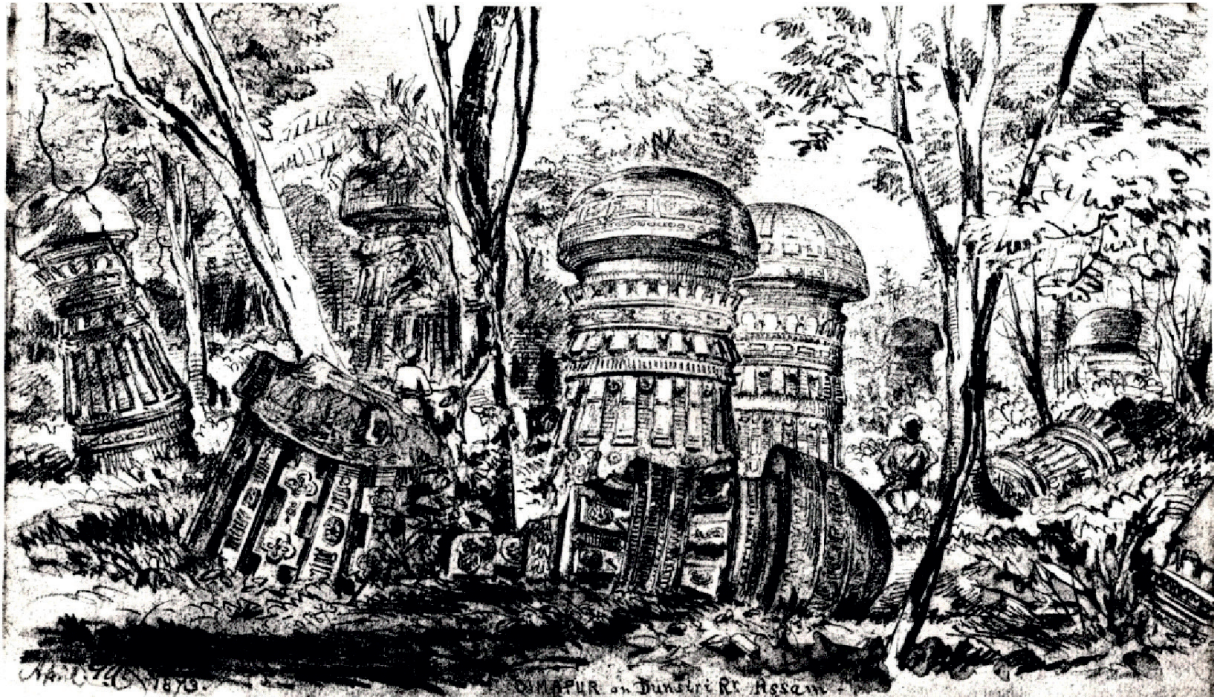
Fig. 1.5: Dilapidated Pillars at Rajbari, Dimapur (Sketch: Godwin-Austen, 1874)
